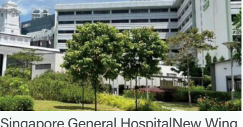
Singapore General Hospital New Wing
